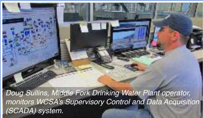
*Doug Sullins, Middle Fork Drinking Water Plant operator, monitors WCSA's Supervisory Control and Data Acquisition (SCADA) system.*
