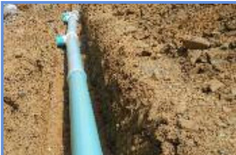
New water line outside Middle Fork Water Treatment Plant.
